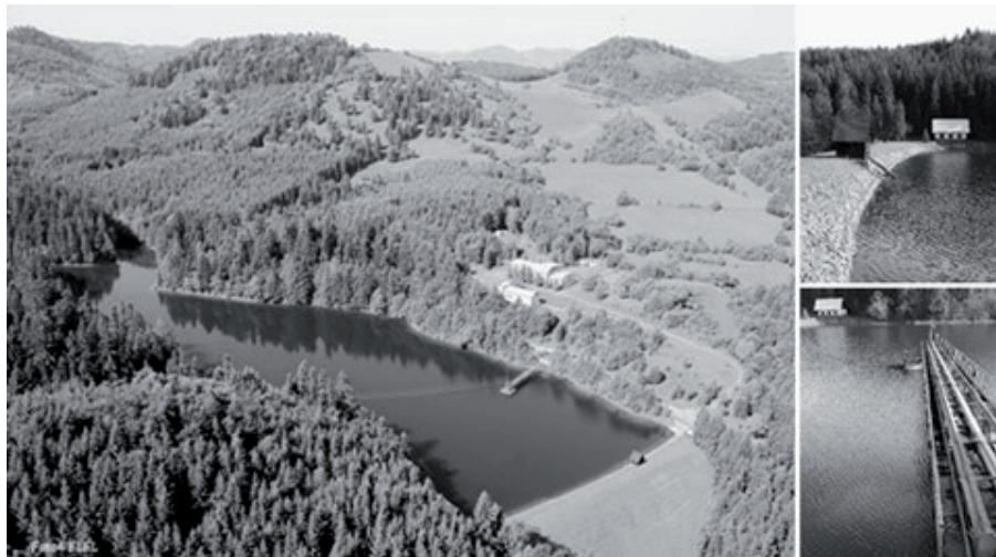
Fig. 2. A view of the Rozgrund water reservoir and the WTP Rozgrund (above the reservoir).
